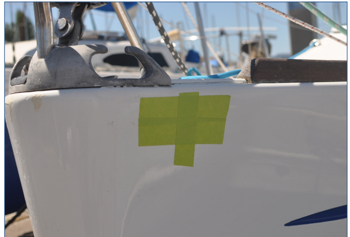
Fig 3: Tape below the deck.
